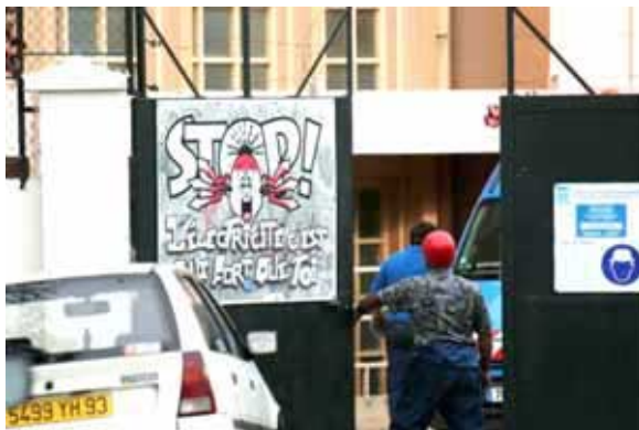
The gate to the sub-station where the boys were electrocuted. The sign says "Stop! Electricity is stronger than you are."
