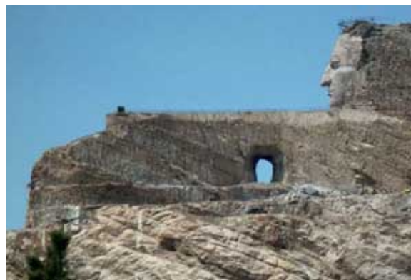
Crazy Hourse monument under construction in the Black Hills.
