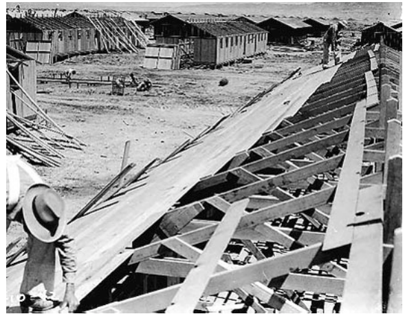
Poston, Arizona, center under construction.
