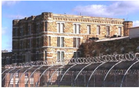
Lansing Correctional Facility. The injection chamber is the corner room on the top floor.
